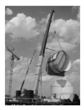
A section of the wind tunnel is lowered into position.
