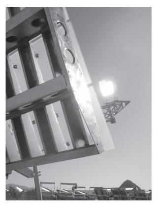
Figure 5: Reflective facets, collector structure, and focused beam in target area
