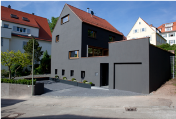
More intensive shades of color are being used on energy-efficient facades. This house in Stuttgart, Germany (built in 1938), was completely renovated with carbon fiber-reinforced ETICS. The insulating system that was used, Carbon DarkSide from Caparol (the market leader in building paints in Germany), offers maximum design possibilities.
